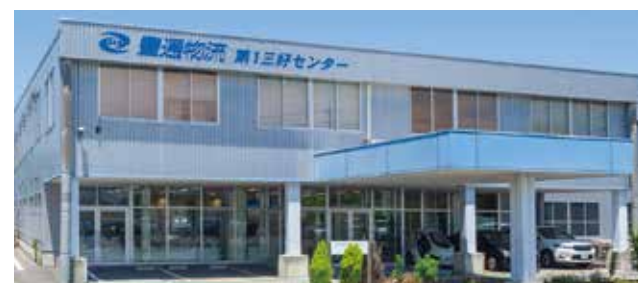
Toyotsu Logistics Service Co., Ltd. (MIYOSHI LOGISTICS CENTER 1)
